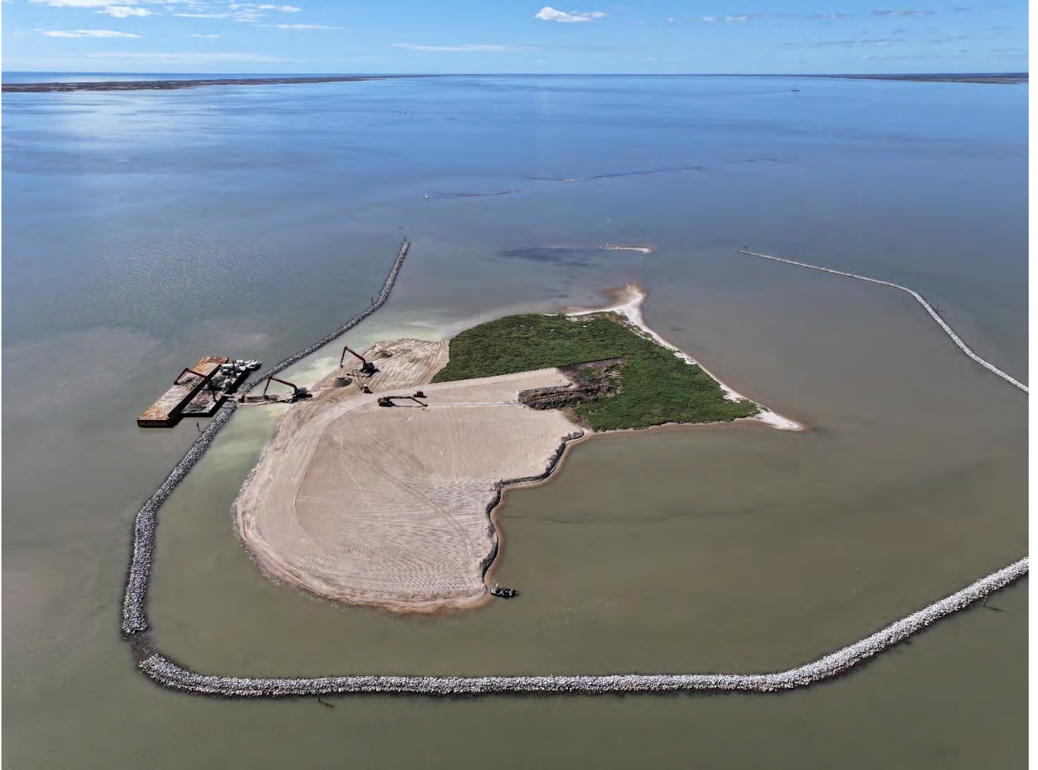
November 5, 2025 Construction Progress.
