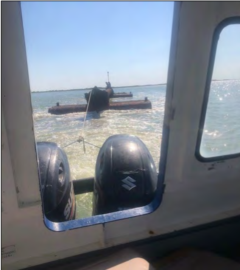
Photo 2. Dredge Pipe Being Removed from Matagorda Island
