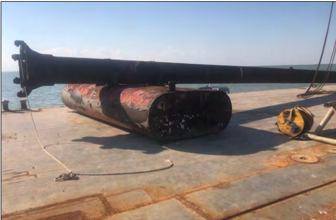
Photo 3. Close up of metal pipe float being removed from Matagorda Island.
