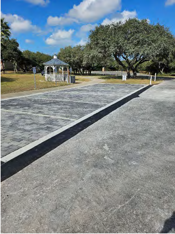
Figure 2 Completed Pavers other end
