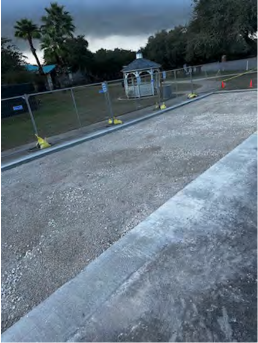
Figure 3 Rock sub-base before paver installation
