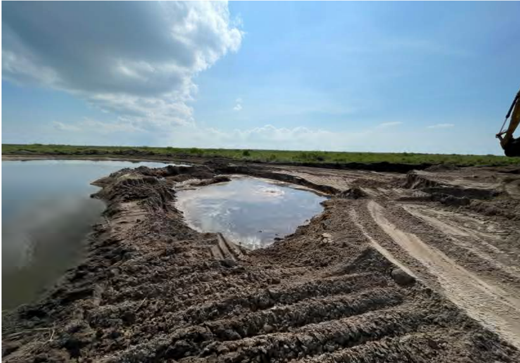
Photo 8. Dig area for reclaimed material for FH-SR-3 breach repair.
