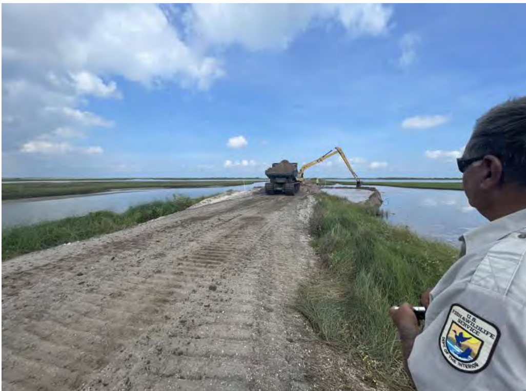
Photo 9. FH-SR-3 breach (caused by Tropical Storm Alberto) repair.
