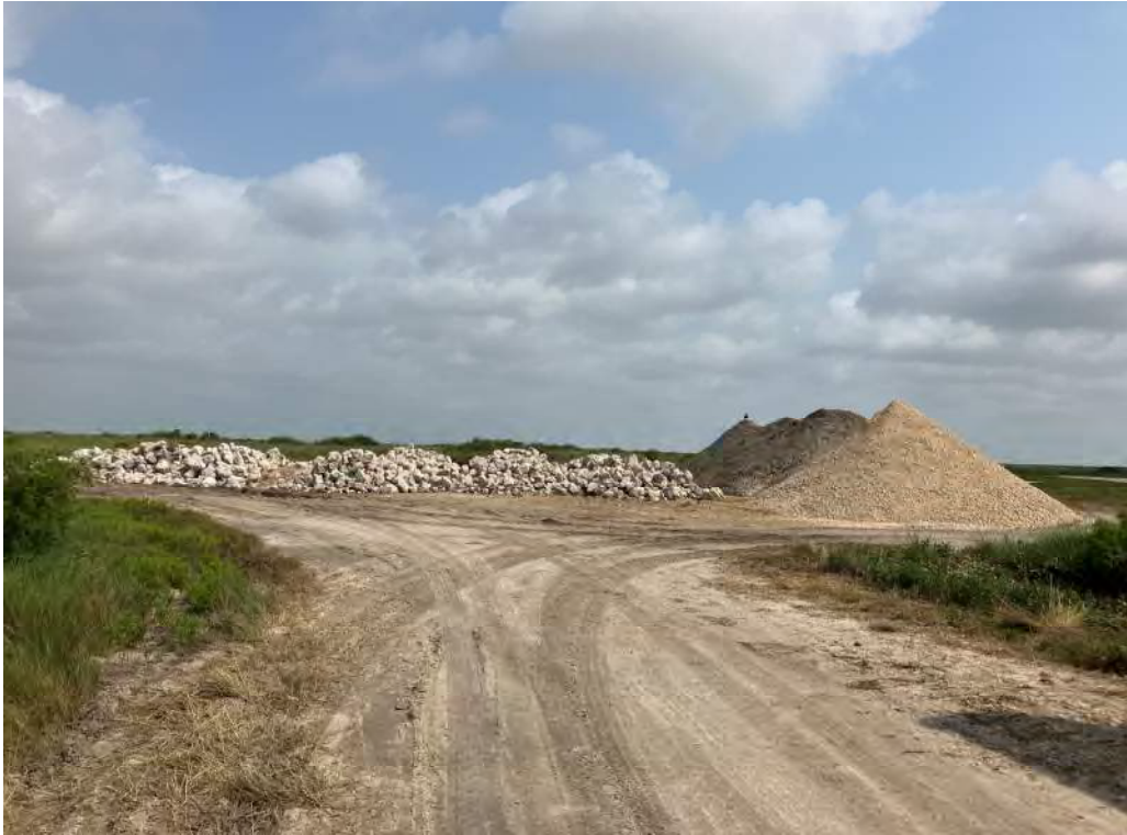
Photo 9. Riprap, road base, and reclaimed material stockpiles near FH-SR-3.
