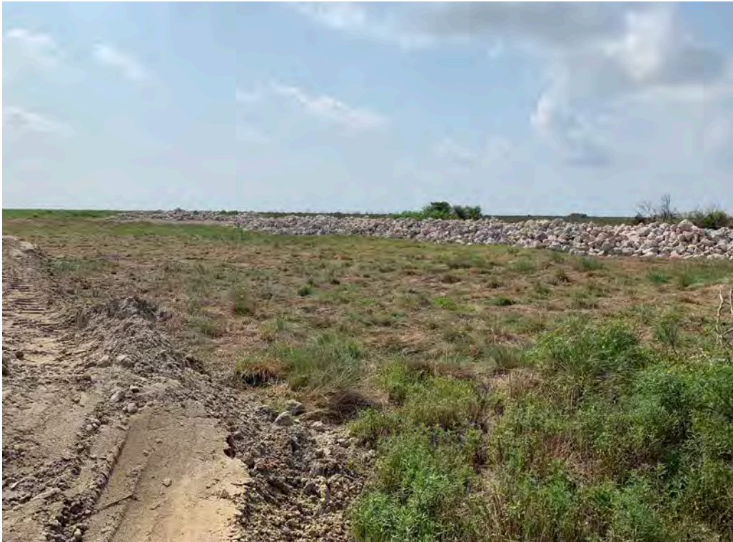
Photo 15. Additional riprap stockpile. Material excavation to extend to approximate edge of stockpile. Contractor as coordinated with USFWS on extents, slopes, etc.
