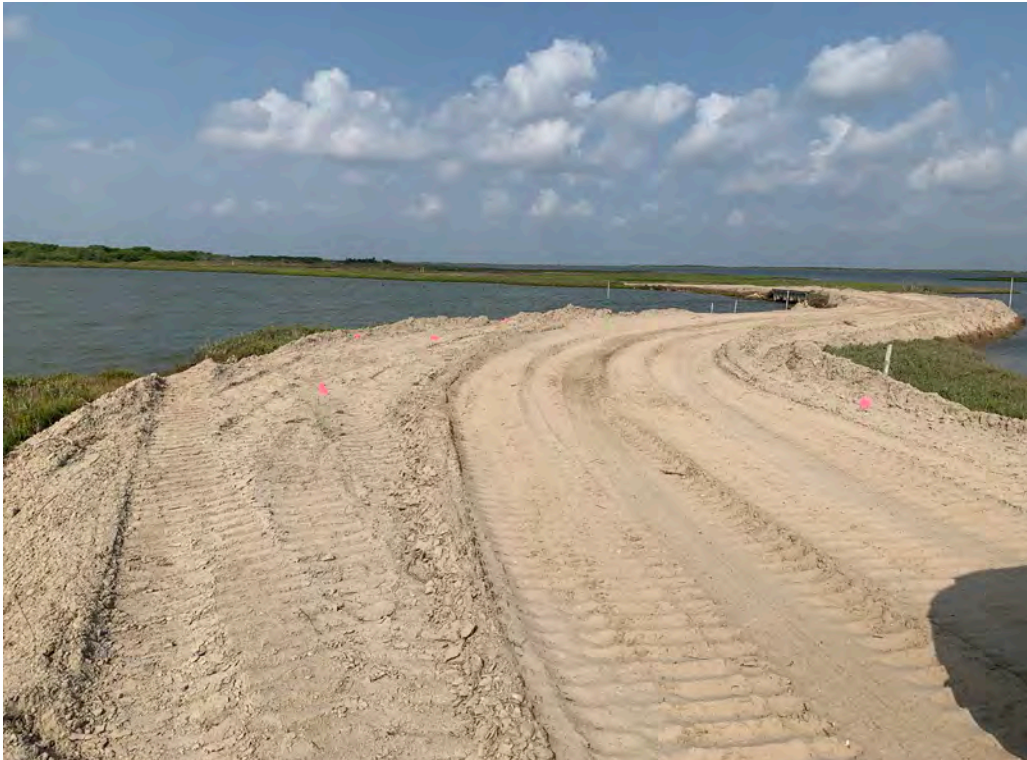
Photo 3. Southern shoreline on eastern end of BC-SR-1 (looking west)
