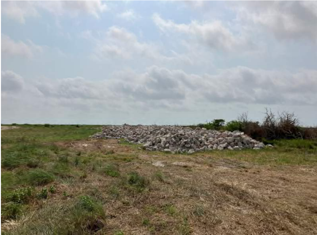
Photo 11. Additional riprap stockpile. Material excavation to extend to approximate edge of stockpile. Contractor as coordinated with USFWS on extents, slopes, etc.
