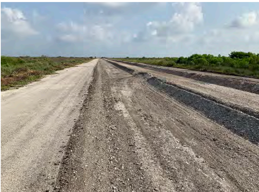
Photo 2. Reclaimed runway material on formed rock stockpile area (looking west)
