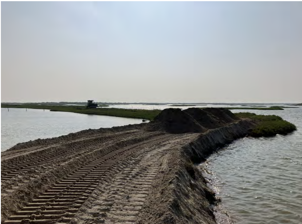
Photo 3. West berm roadway approach of BC-SR-1 site material (looking east)
