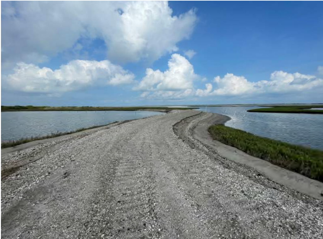
Photo 6. Roadway heading towards BC-SR-1 (facing west)
