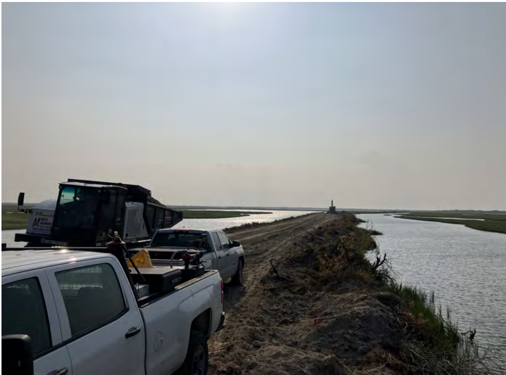
Photo 1. Roadway section northwest of B-SR-1 (looking southeast)
