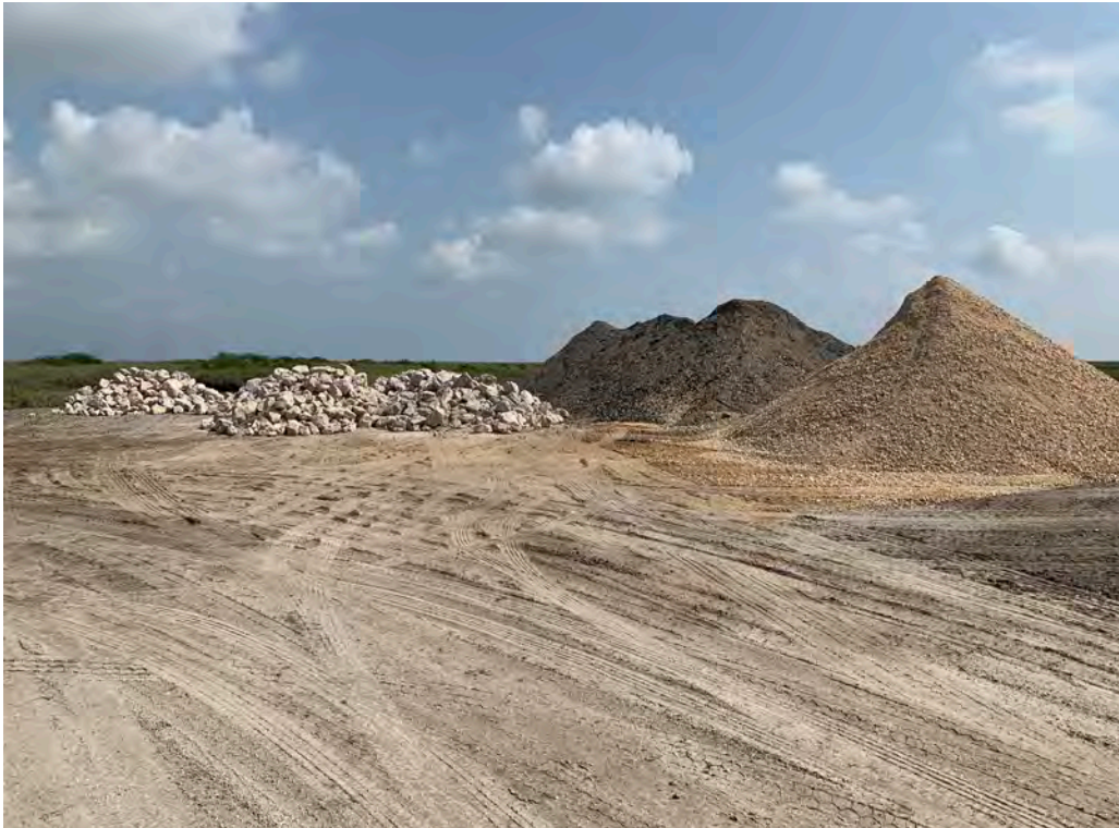
Photo 13. Riprap, road base, and reclaimed material stockpiles near FH-SR-3.
