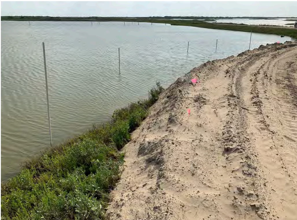
Photo 9. North side of breach repair at BC-SR-1 (looking east).
