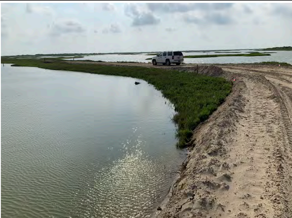
Photo 10. North side of breach repair at BC-SR-1 (looking east).
