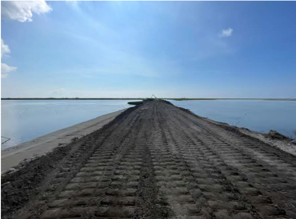
Photo 12. FH-SR-3 (facing east)
