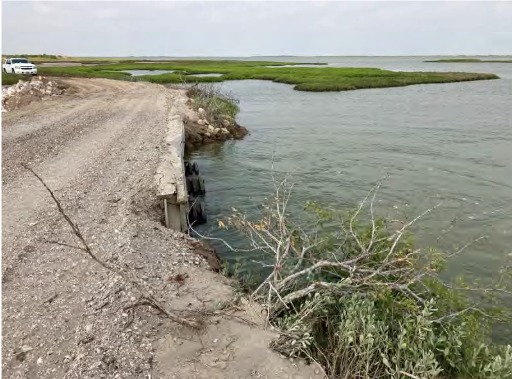
Photo 5. Northern shoreline of BC-SR-1 at existing culvert location (looking west).
