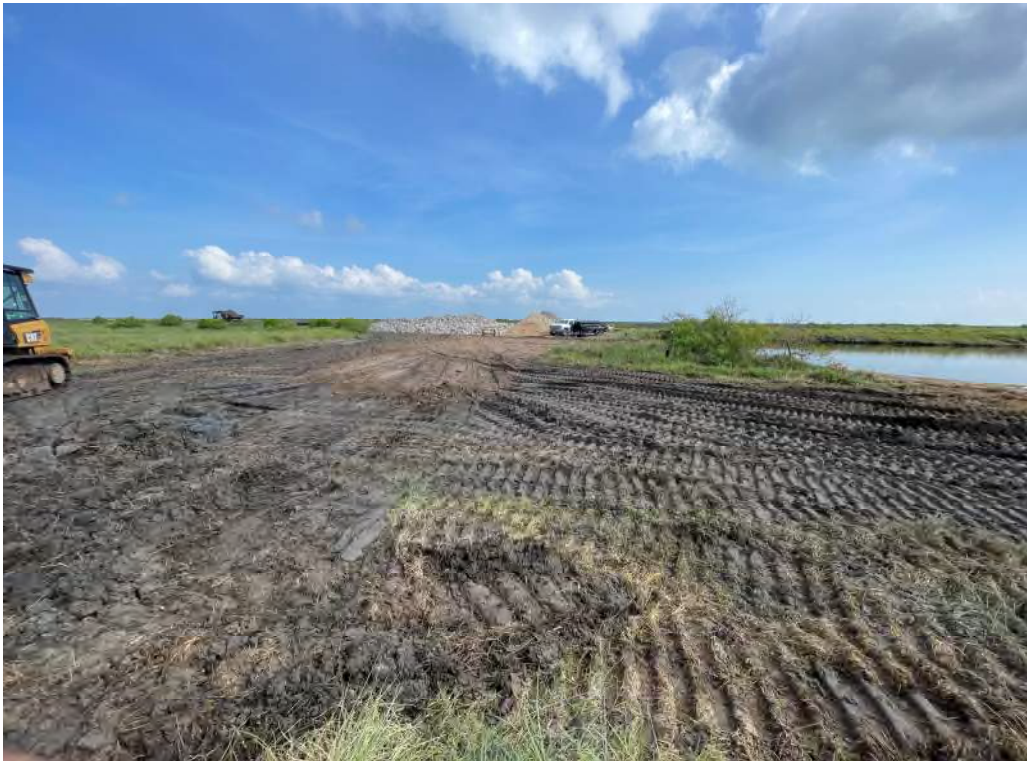
Photo 7. Riprap, base and reclaimed material near FH-SR-3
