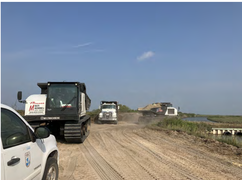
Photo 2. Roadway section northwest of B-SR-1 (looking northwest)
