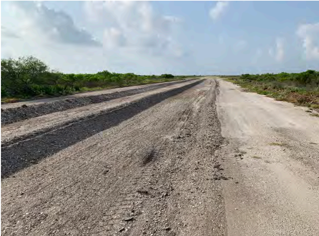
Photo 1. Reclaimed runway material on formed rock stockpile area (looking east)
