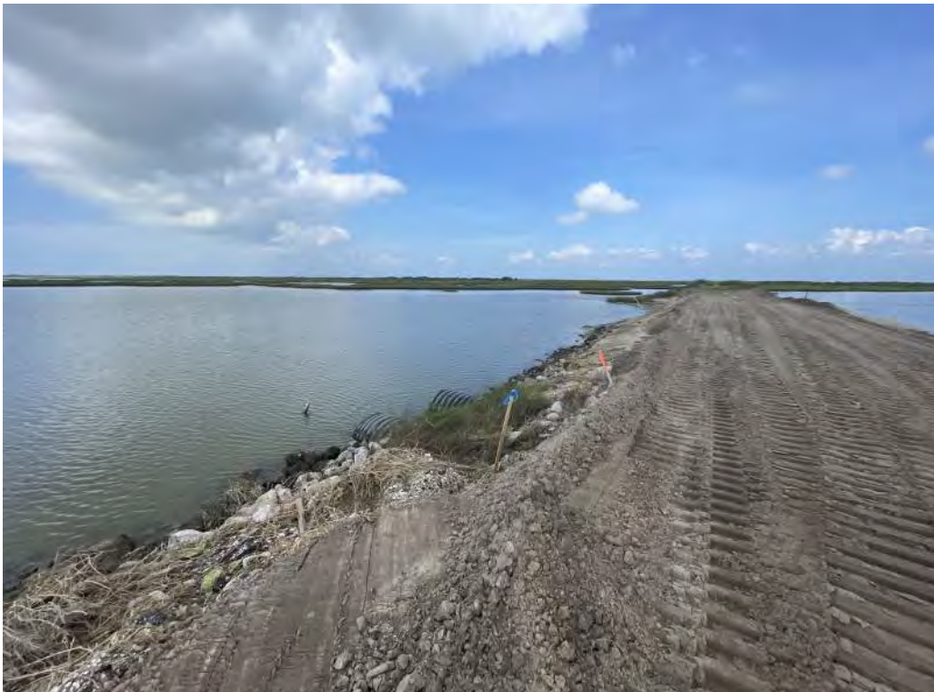
Photo 11. Middle of FH-SR-3 (facing west)
