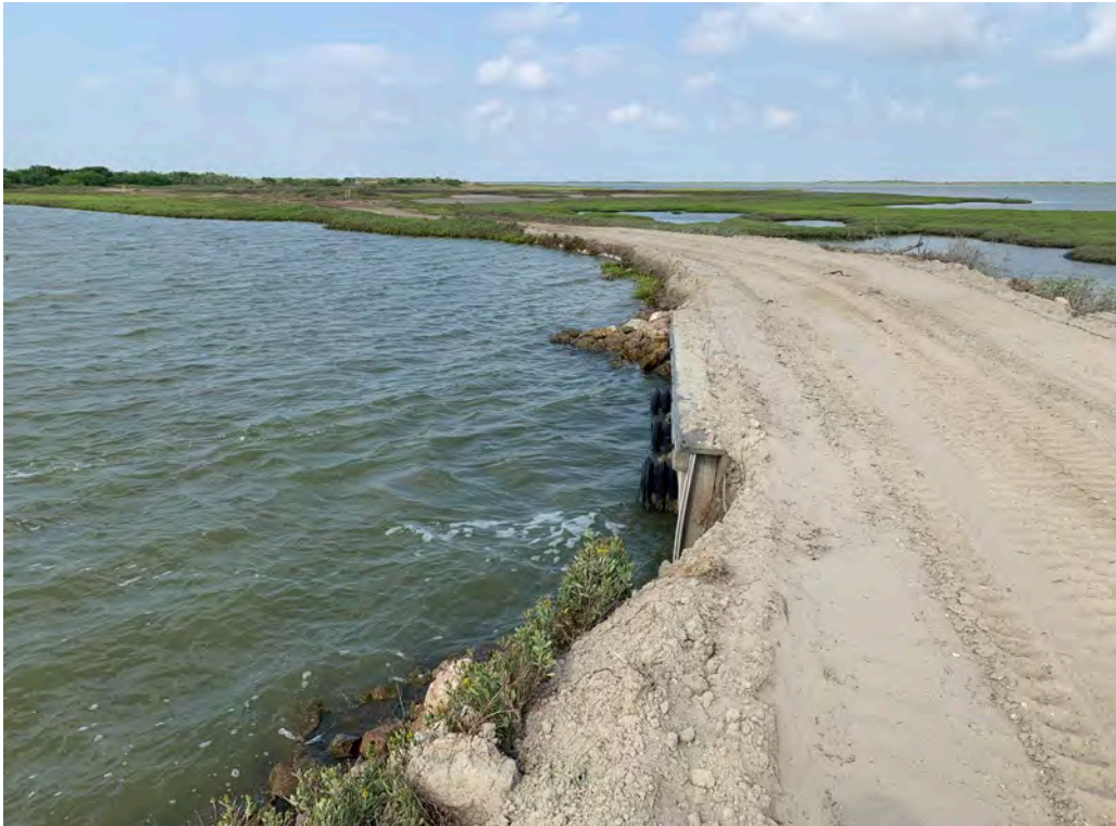
Photo 7. Existing culverts on south side of BC-SR-1.
