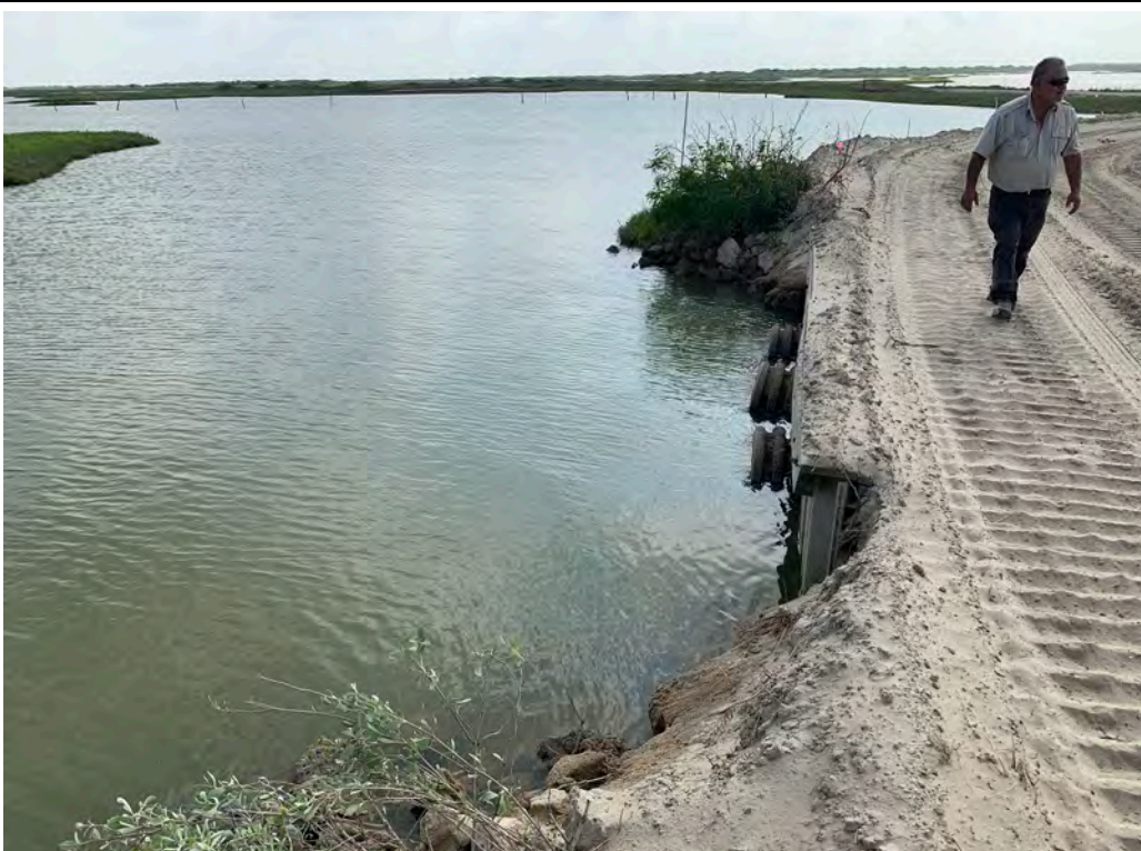
Photo 8. Existing culverts on north side of BC-SR-1.
