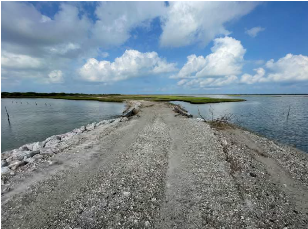
Photo 4. BC-SR-1 (looking west)
