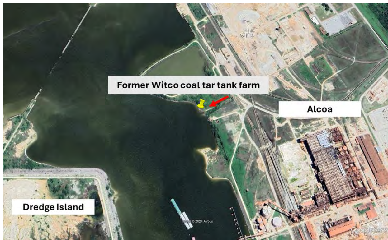
Figure 3. Sediment core collection location (yellow pin) where the drainage area next to the slurry wall enters Lavaca Bay. The red arrow shows the location of the slurry wall and direction of runoff from land.
