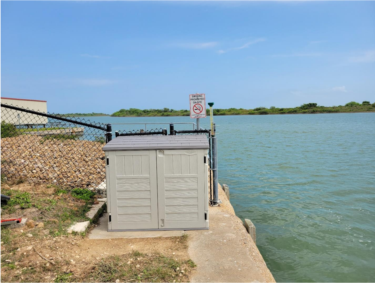
Figure 1. Shed that has been constructed to house the FlowCytobot at the TPWD's Port O'Connor facility.
