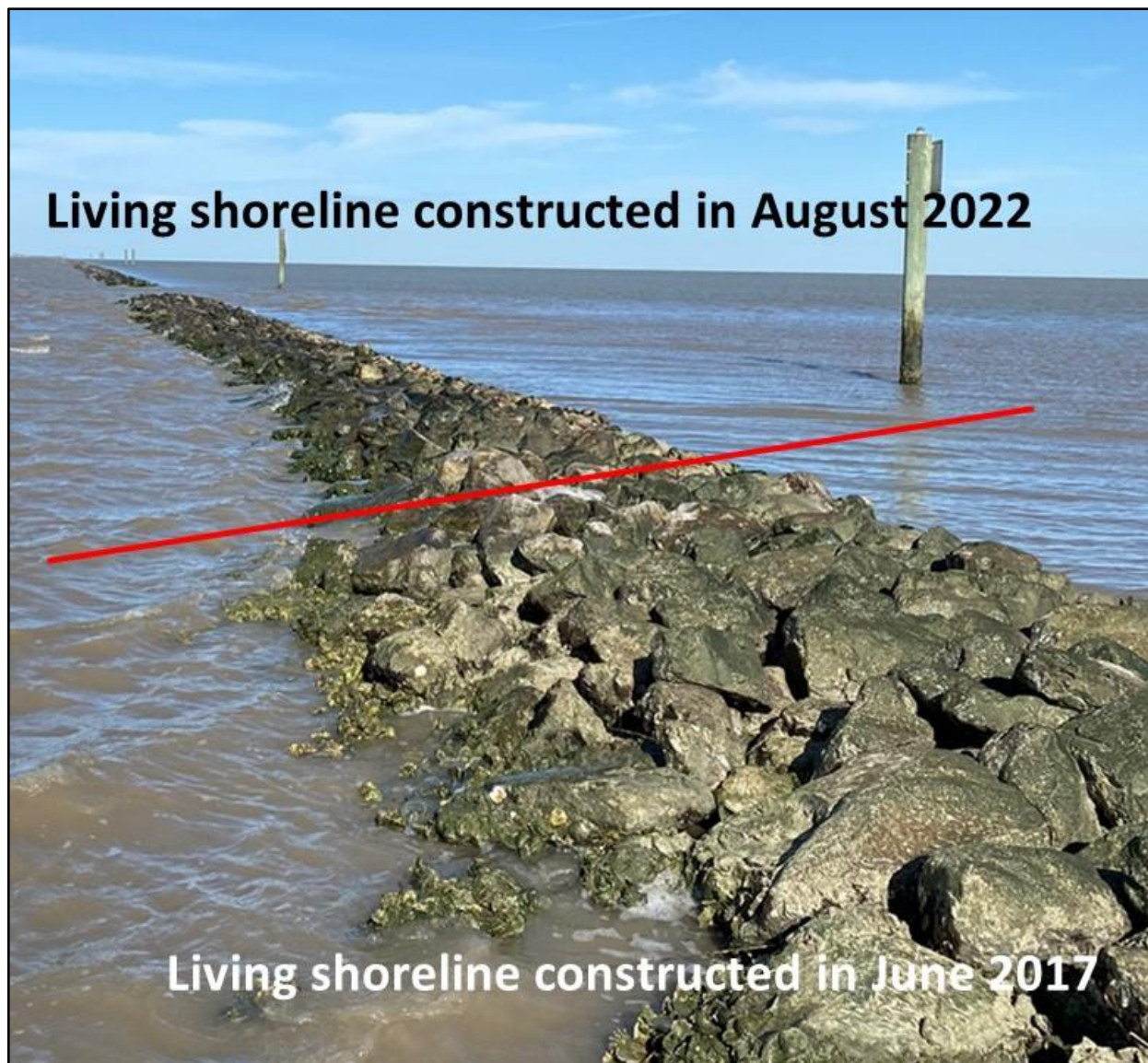
Figure 4. Schicke Point living shoreline where the portion constructed in August 2022 (above the red line) connects to the portion constructed in June 2017 (below the red line). Note oysters colonizing the older reach of living shoreline. Photo taken March 17, 2023 by FNI.
