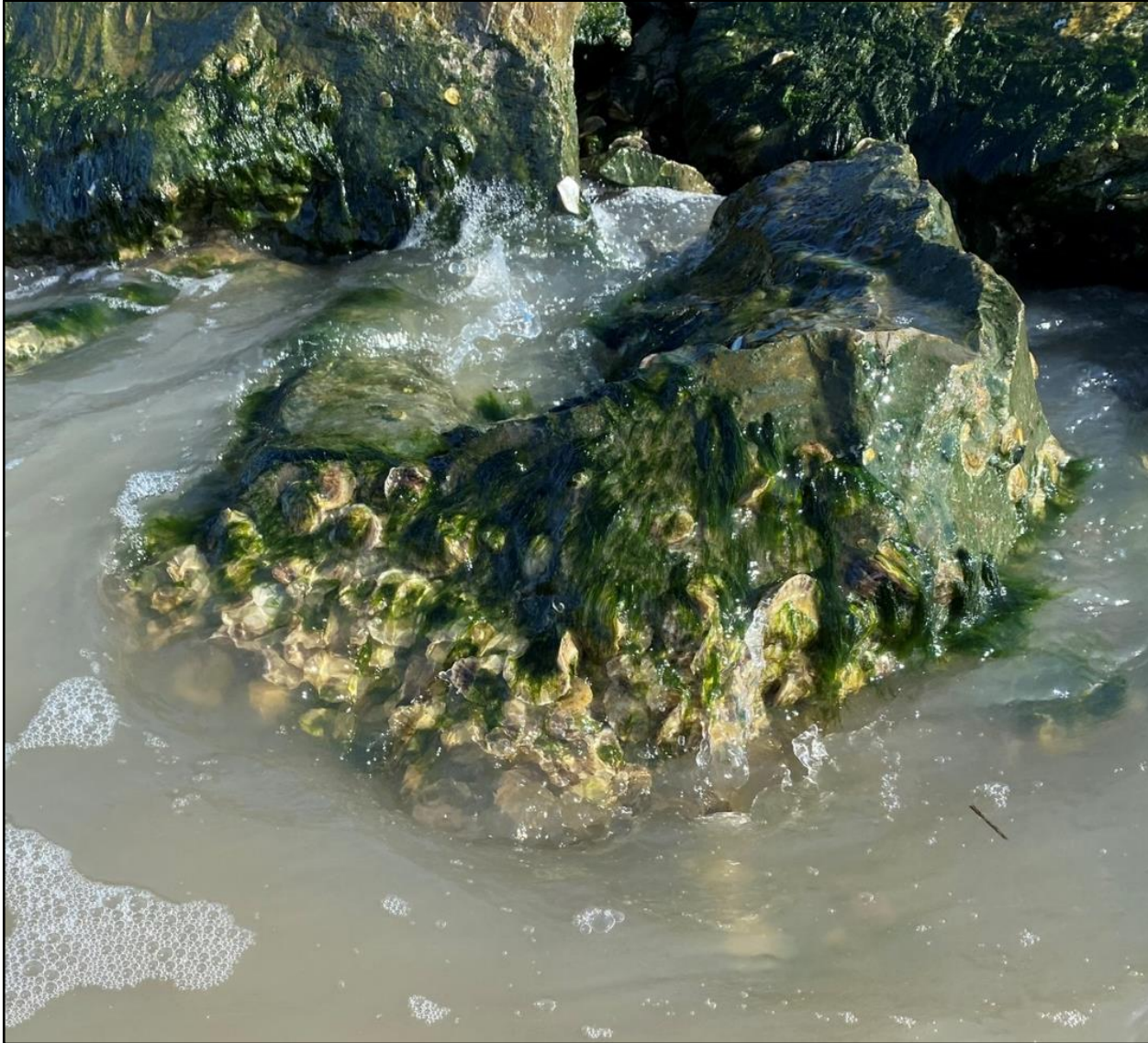
Figure 2. Shore-facing rocks of Schicke Point living shoreline constructed in August 2022 demonstrating oyster colonization. Photo taken by FNI on March 17, 2023.
