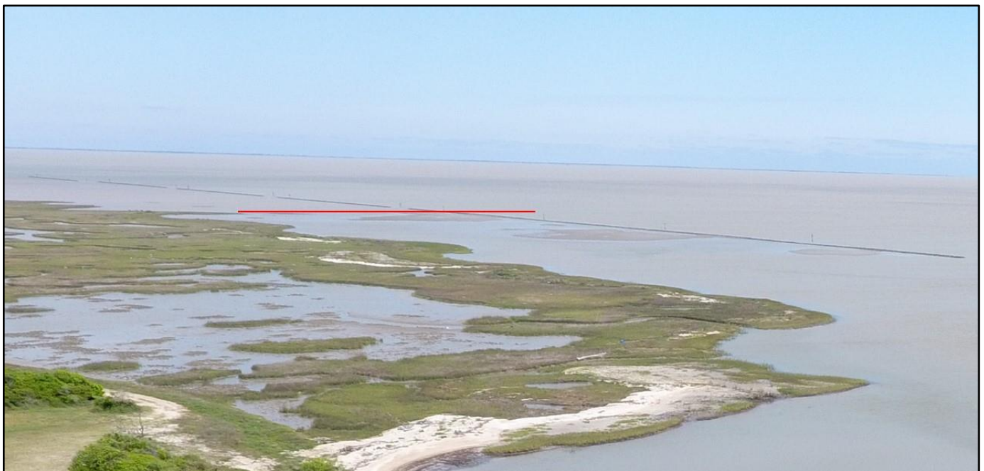
Figure 6. Schicke Point living shoreline where the portion constructed in August 2022 (above the red line) connects to the portion constructed in June 2017 (below the red line). Note sediment accumulated behind the older reach of living shoreline. Photo taken March 17, 2023 by FNI.
