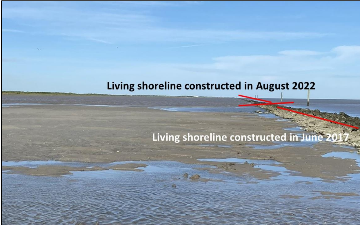
Figure 5. Schicke Point living shoreline where the portion constructed in August 2022 (above the red line) connects to the portion constructed in June 2017 (below the red line). Note sediment accumulated behind the older reach of living shoreline. Photo taken March 17, 2023 by FNI.
